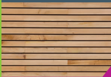
Typical Timber Façade
