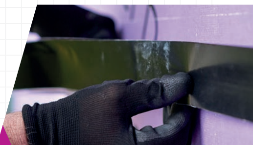
Weather Defence Joint Tape being applied
